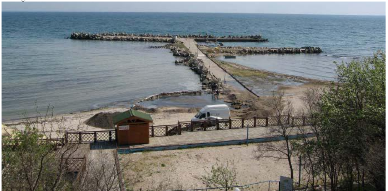
Many similar structures can be found along the Bulgarian coast, all dating from the same period (1960s to 1980s).
